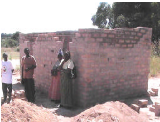
Construction of the Caretaker's house in progress.
