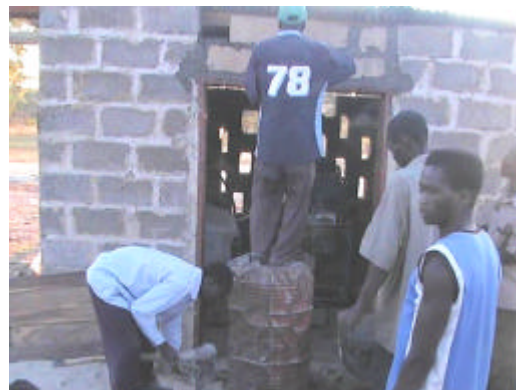
The hammermill house being worked on
