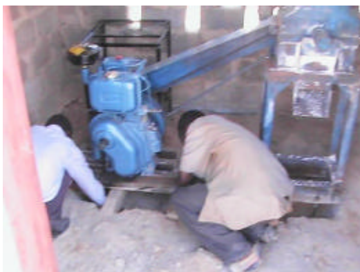
HM being installed after trials and demonstration.
