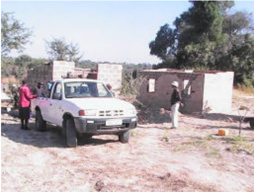
Materials and Hammermill being delivered
